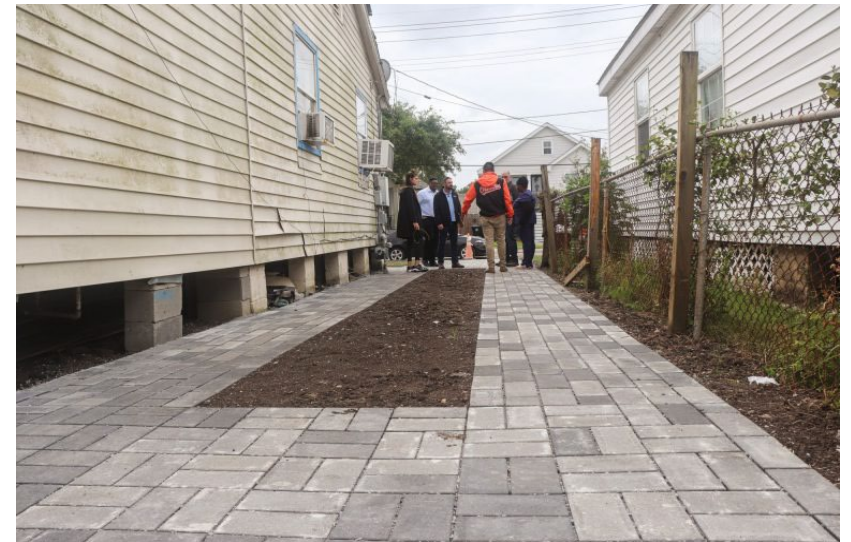
Thrive New Orleans remade a concrete driveway with permeable pavers. ( Source: Thrive New Orleans from Kresge )
